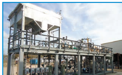
Hydrogenation Skid Module
