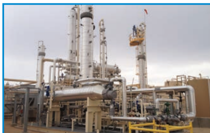
30 MMSCFD Natural Gas Processing Plant, Goldsmith, TX
