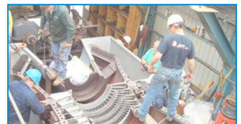
Siemens Westinghouse 251B Gas Turbine Major Overhaul
