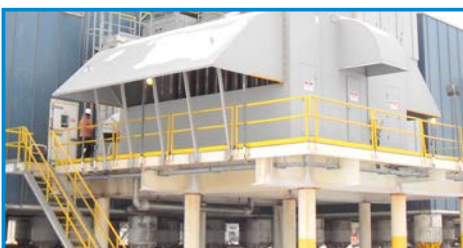
Filter House with Inertial Separators, Prodhoe Bay, Alaska
