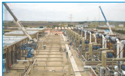
69,000 HP (9) Compressor Station
