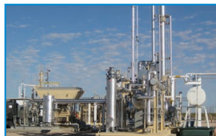
1.3 MMSCFD Natural Gas Processing Plant, Mentone, TX
