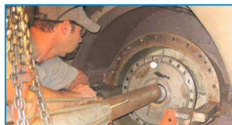
GE Frame 5 Turbine Rotor Alignment
